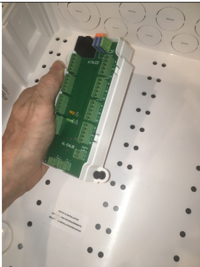
Preparing to install
