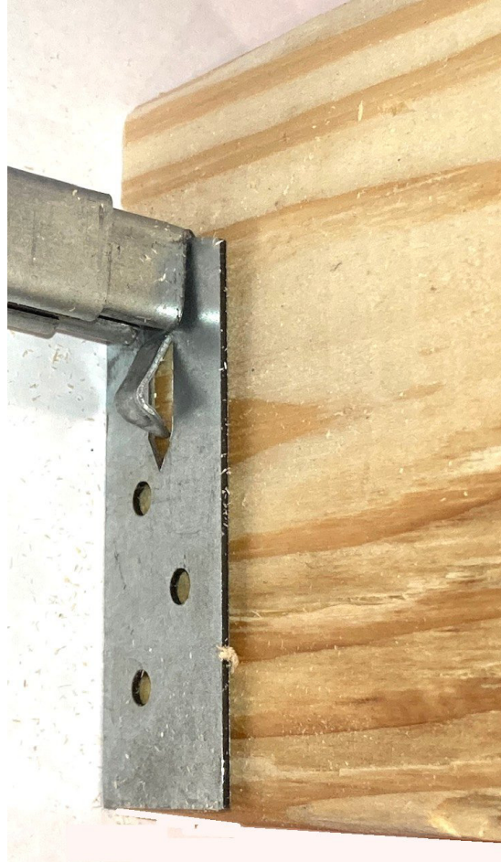
Beam installation
